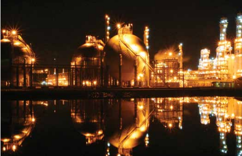
▲ High pressure gas storage vessels.
